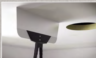
E / Check joints and centre of panels
