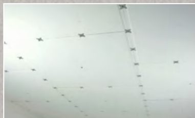
B / Panel installation Fix the Rockfon Mono Acoustic panels to the grid. Direct installation (mechanical / adhesive) on airtight substrate is also possible.
